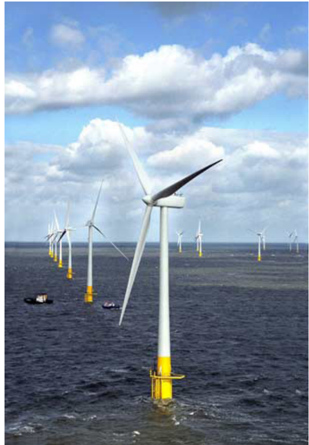
Source: Wikipedia Thanet offshore turbines
