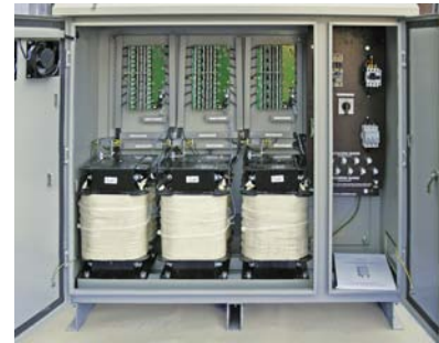
Internal view of a Sollatek Outdoor Isolating AVR.
