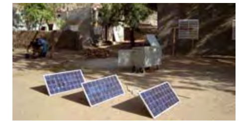
Mobile solar powered unit
