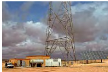
Remote communication site powered by Sollatek Solar
