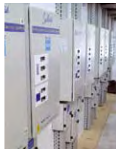
Sollatek SCCs controlling the system
