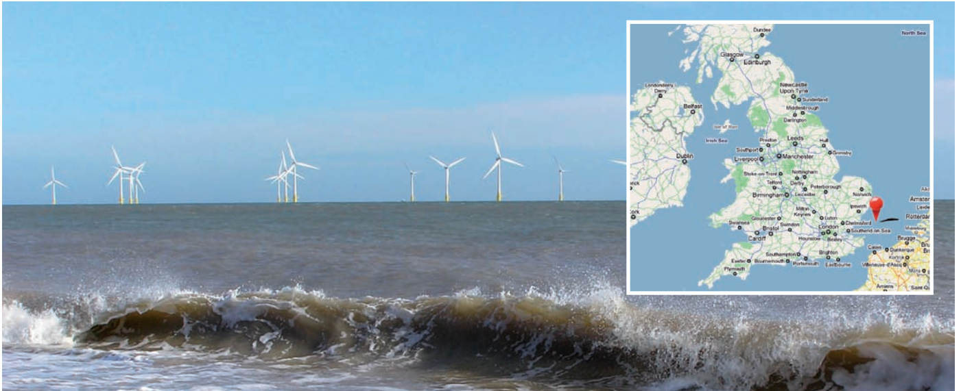
Source: SSE RWE, Greater Gabbard offshore turbines
