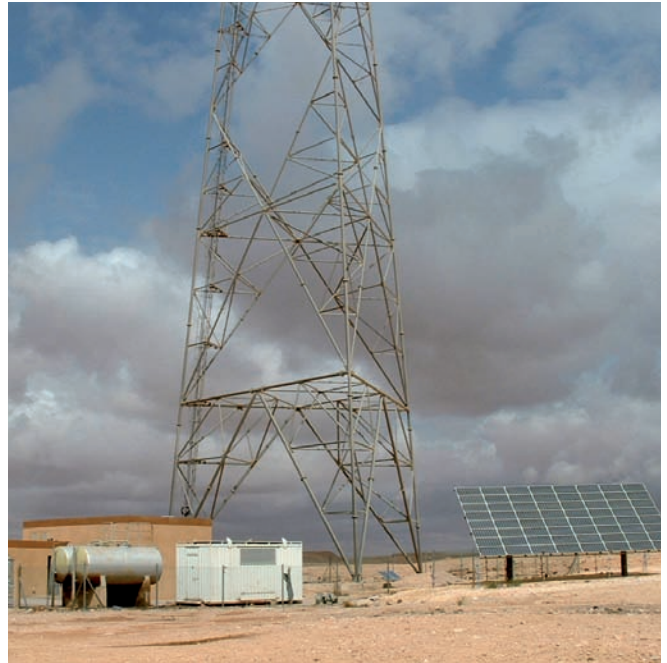
BTS site using PV solar power instead of redundant diesel generator
