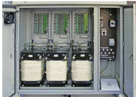
Internal view of a Sollatek Outdoor Isolating AVR.
