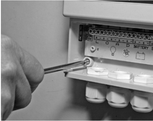
Figure 11: Fixing the SPCC10 to the wall
