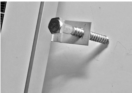
Figure 3: Fixing the solar module to the ceiling using the supplied coach screw
