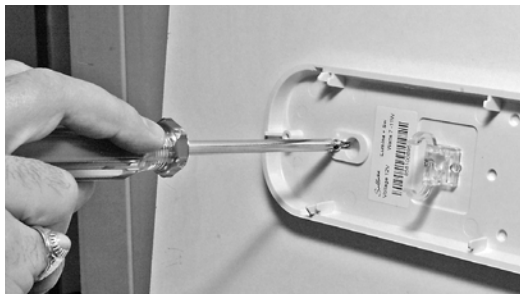
Figure 8: Attaching Lumina to wall
