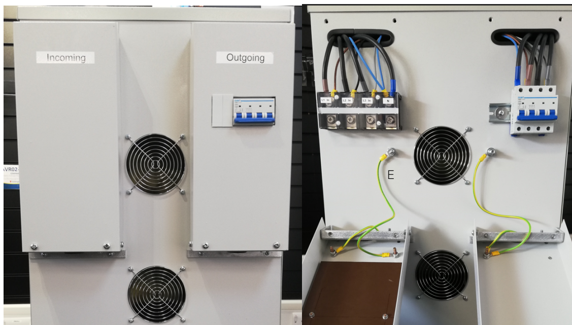
Fig 4.6. AVR site connections
